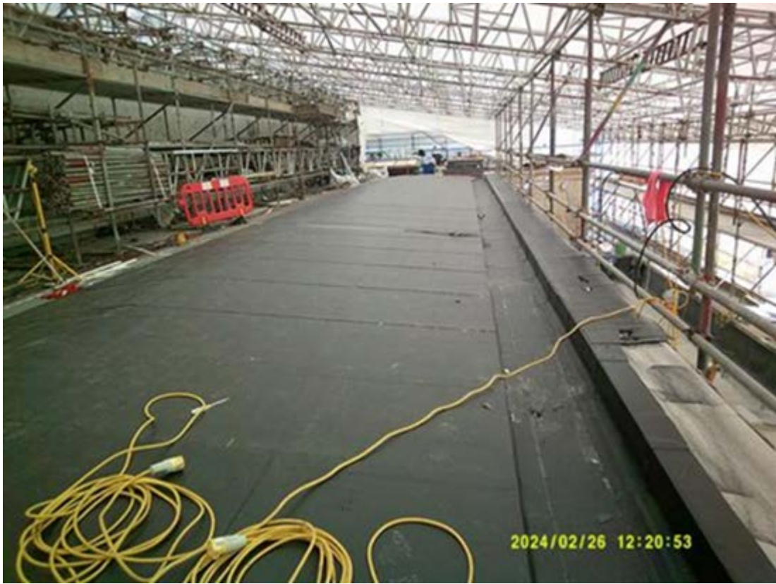
Image 3 ROOF 5 - NEW ROOF COVERING WORK IN PROGRESS
