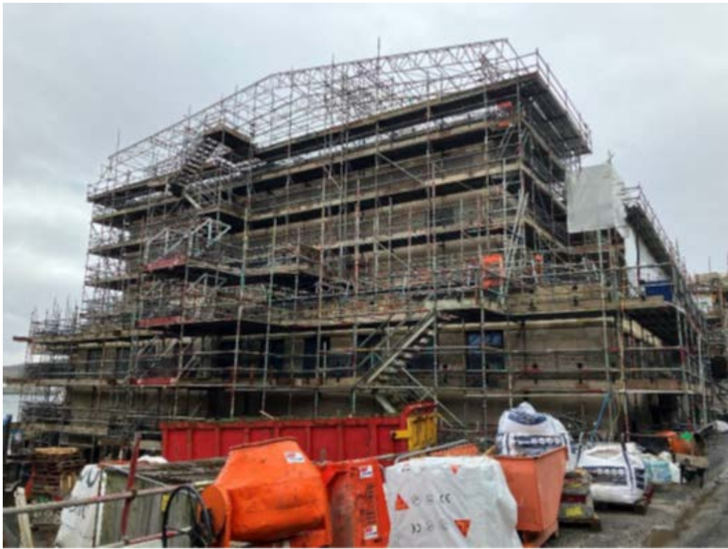
Image 5 FLYTOWER VIEWED FROM MACKINLAY STREET - TEMPORARY SCAFFOLD AND ROOF TRUSSES INSITU.
