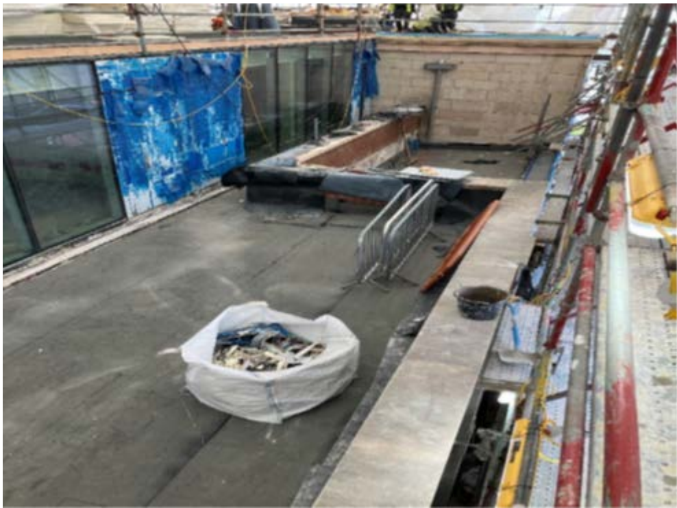
Image 4 ROOF 4 - OVERVIEW OF FIRST FLOOR OFFICES LOOKING EAST
