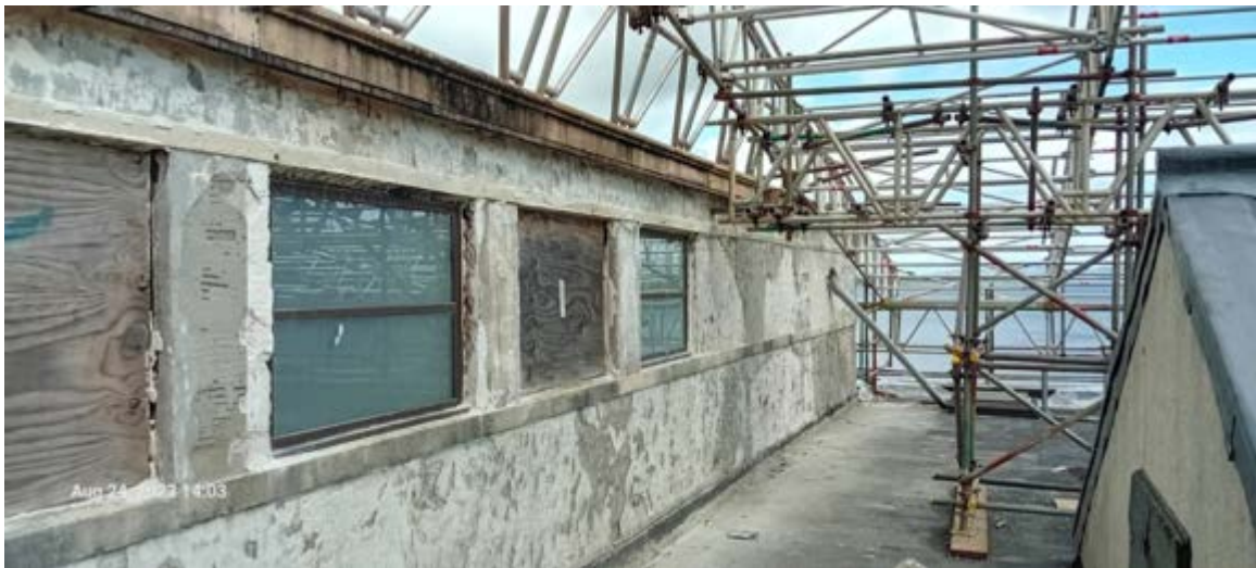
Image 29 SOUTH FACE OF FLY-TOWER FOLLOWING RENDER REMOVAL WORKS.
