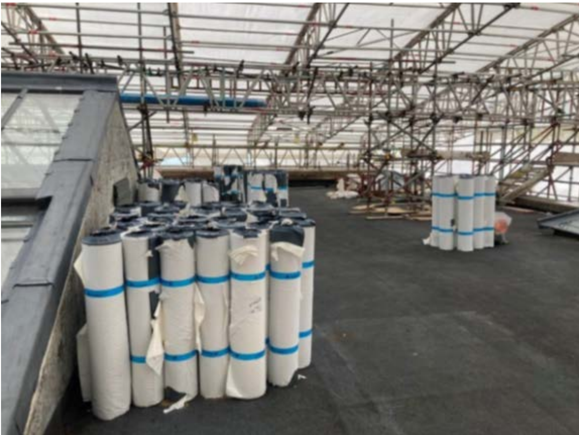
Image 25 MAIN ROOF: ROOFING MATERIALS STORED ON SITE.
