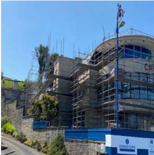
Image 34 PHOTO 1 - SOUTH AND EAST ELEVATIONS: SCAFFOLDING INSITU.
