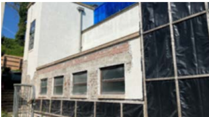
Image 37 REMOVAL OF RENDER TO SOUTH ELEVATION HAS STARTED EXPOSING BRICKWORK.
