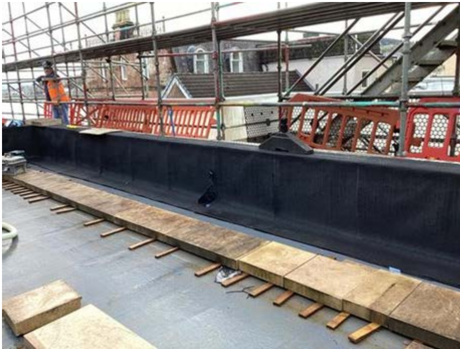
Image 22 SOUTH ELEVATION COPES REMOVED TO ALLOW INSTALLATION OF ROOF COVERING MEMBRANE.
