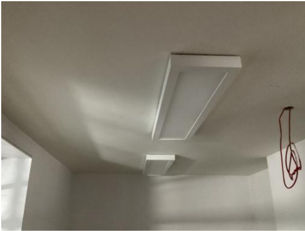
Image 18 LIGHT FITTINGS INSTALLED IN CARETAKERS HOUSE.
