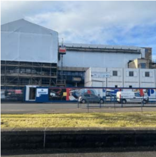
Image 14 ROOF 3B TEMPORARY ROOF FRAME AND SHEETING INSITU.
