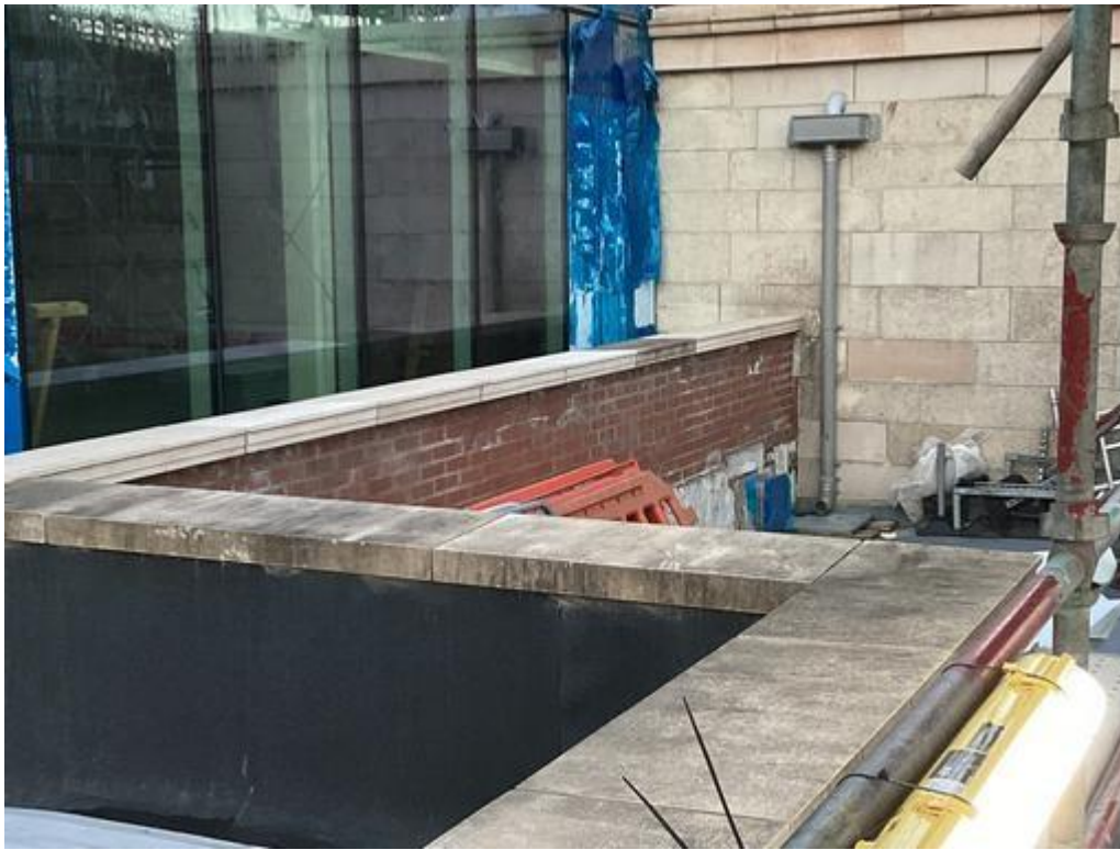
Image 11 SOUTH ELEVATION: COPING REINSTALLED ALONG ROOF 4.
