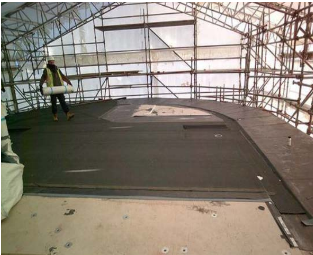
Image 7 ROOF 3B FRONT ROTUNDA- NEW ROOF MEMBRANE BEING FINALISED.
