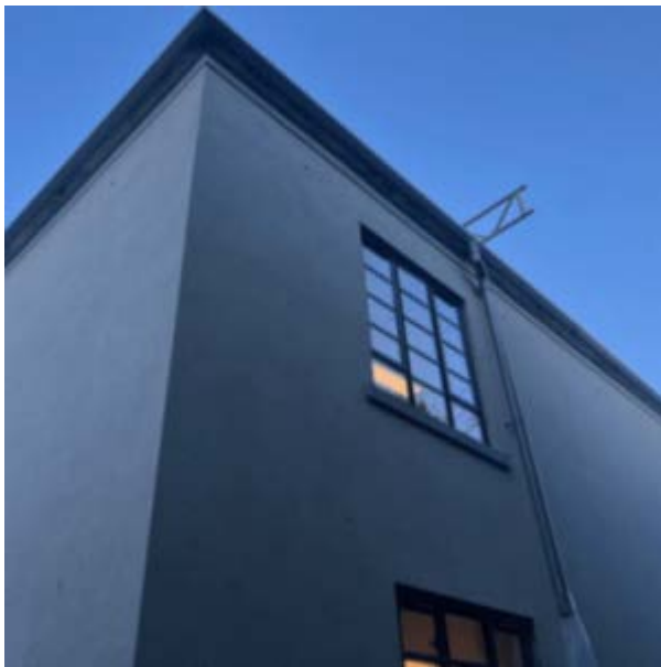
Image 12 CARETAKERS HOUSE: SOUTH ELEVATION SHOWING GOOD QUALITY OF NEW RENDER FINISH.
