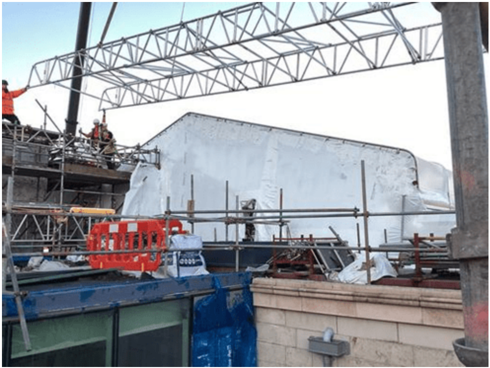
Image 16 ROOF 5:1ST FLOOR OFFICE SUITE: ASSEMBLY OF TEMPORARY ROOF STRUCTURE.
