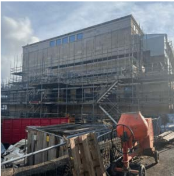
Image 15 ROOFS 2B, 2C AND 2D ERECTION OF SCAFFOLD AND TEMPORARY ROOF
