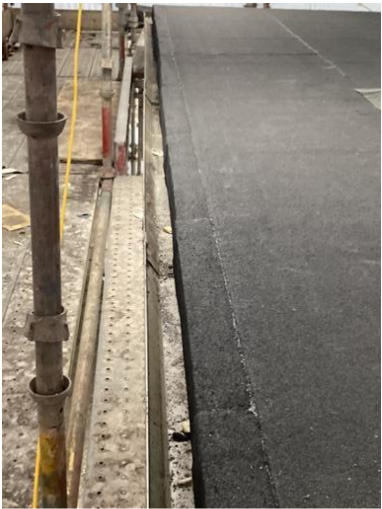
Image 17 CARETAKERS HOUSE: PERIMETER GUTTER INSTALLED.
