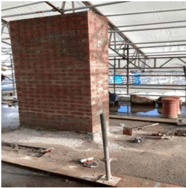
Image 20 CARETAKERS HOUSE CHIMNEY. REBUILT.
