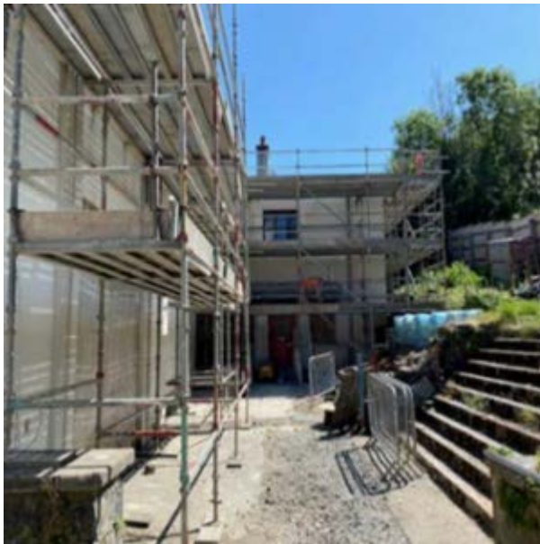
Image 35 PHOTO 2 - WEST ELEVATION: SCAFFOLD
