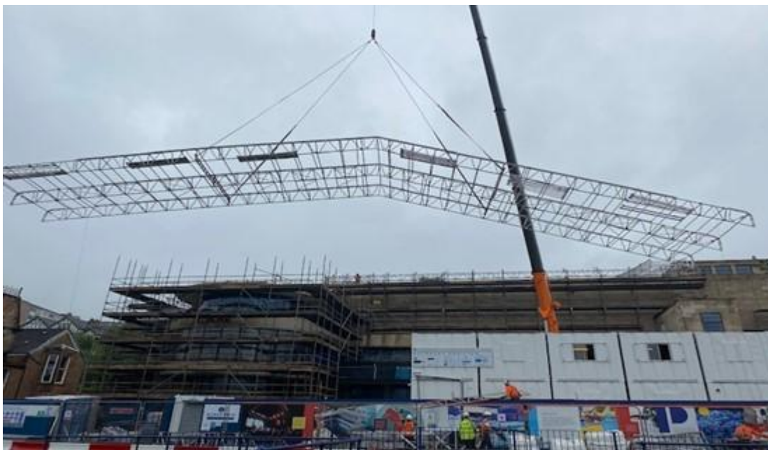
Image 32 TEMPORARY ROOF FRAME BEING LIFTED INTO POSITION
